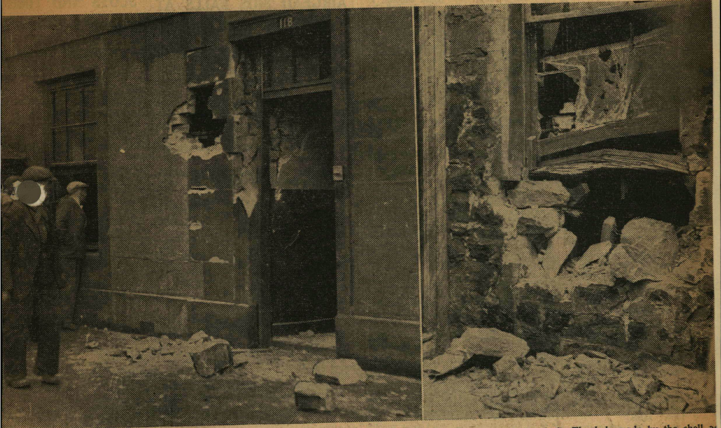
This is what happened to a house in Salamander Street, Leith, when it was hit to-day by a 100lb. dummy shell. Left—The hole made by the shell as it entered the house. Right—The havoc created by its exit.
