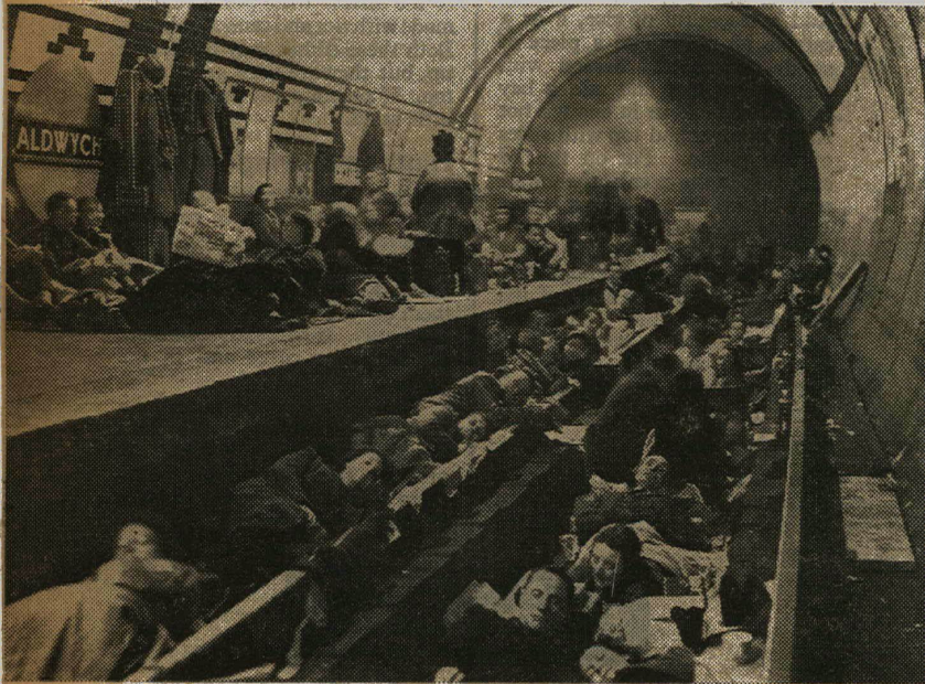
Londoners sleeping on the platforms and between the rails at Aldwych tube station which has been turned into a refuge.
