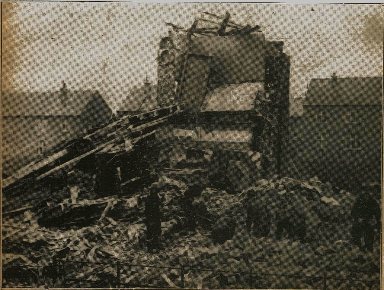
Members of the demolition squad at work amid the wreckage of houses struck by a bomb in the Edinburgh area last night. An eight-years-old boy and his little sister were killed.
